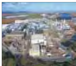
Kemsley Paper Mill could get another power station built
